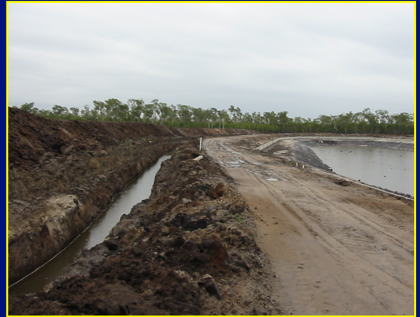
Recharge trench constructed around the perimeter of the dewatered excavation
