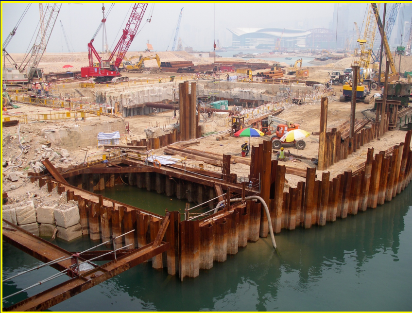
Dry Excavation Sheet Piling
