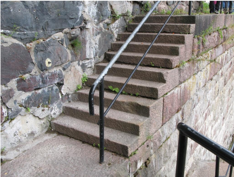
Figure 12. Wall and stairs made of quarried stone in the Suomenlinna dry docks. The wall on the left is made of boulders collected from nearby areas.
