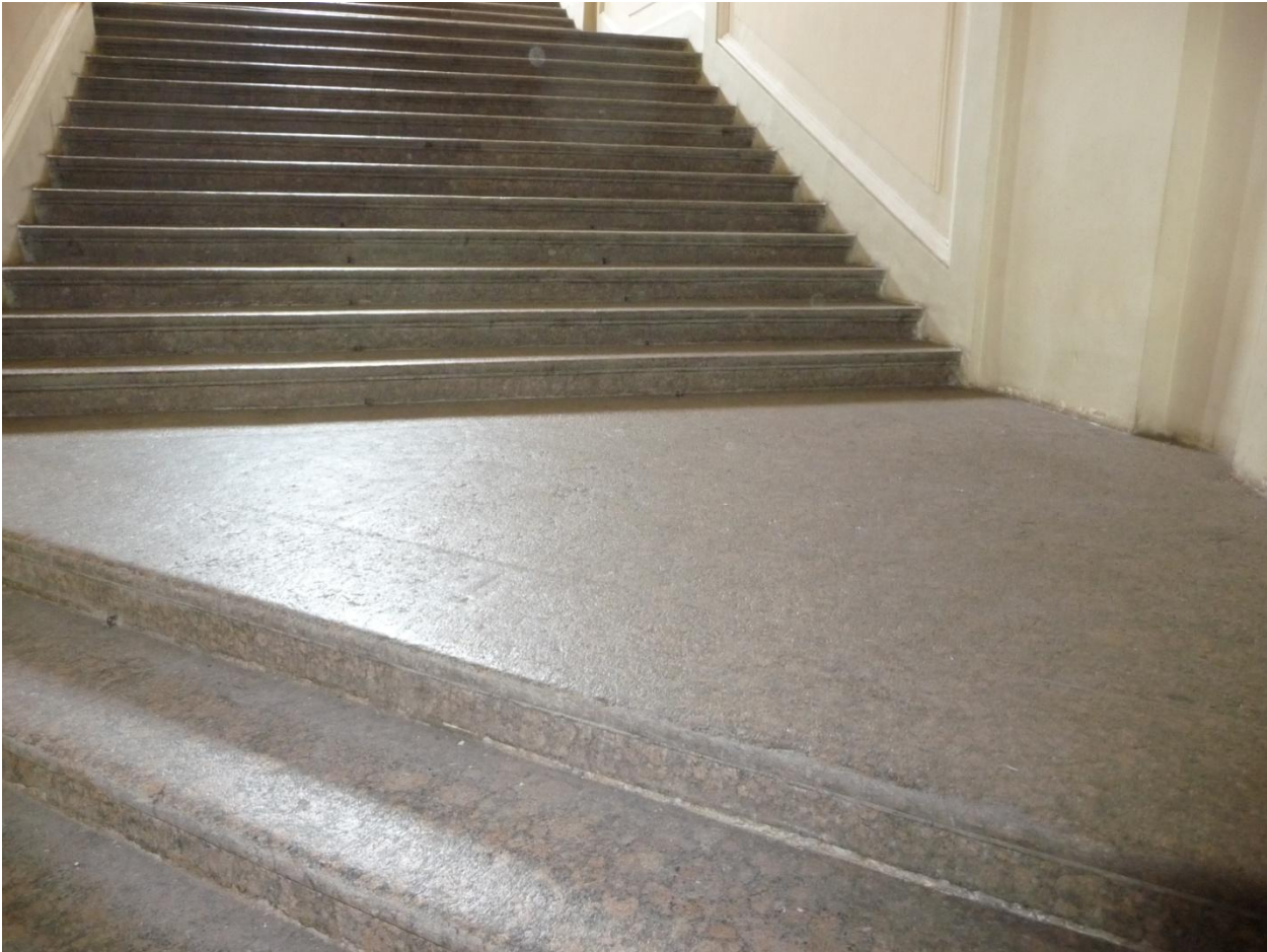
Figure 127 View of the stairs of the academy of arts done in monolithic steps of rapakivi granite
