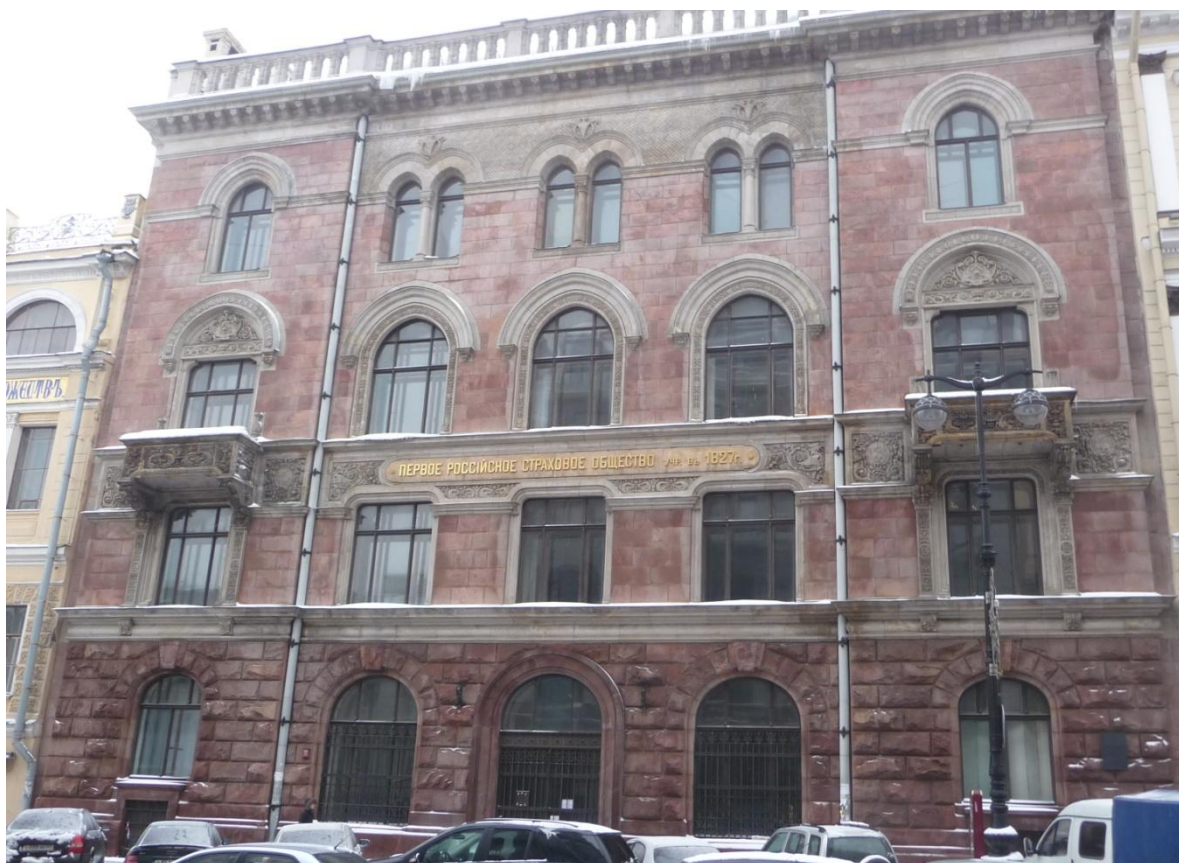
Figure 44 Building of the first Russian Insurance Company made of sandstone
