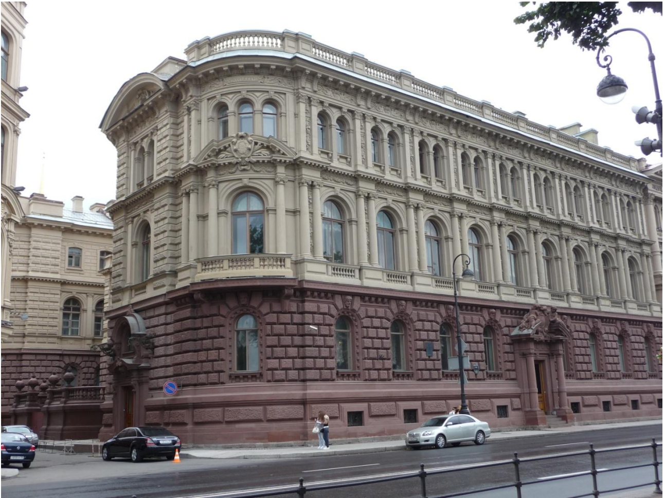
Figure 81 View of the Grand Duke Michail Michailovich's Palace with rapakivi granite basement
