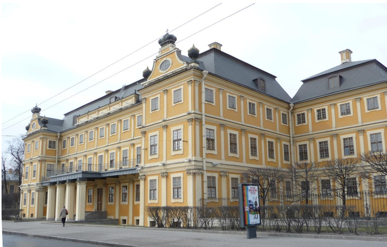
Figure 133 View of the Menshikov's house
