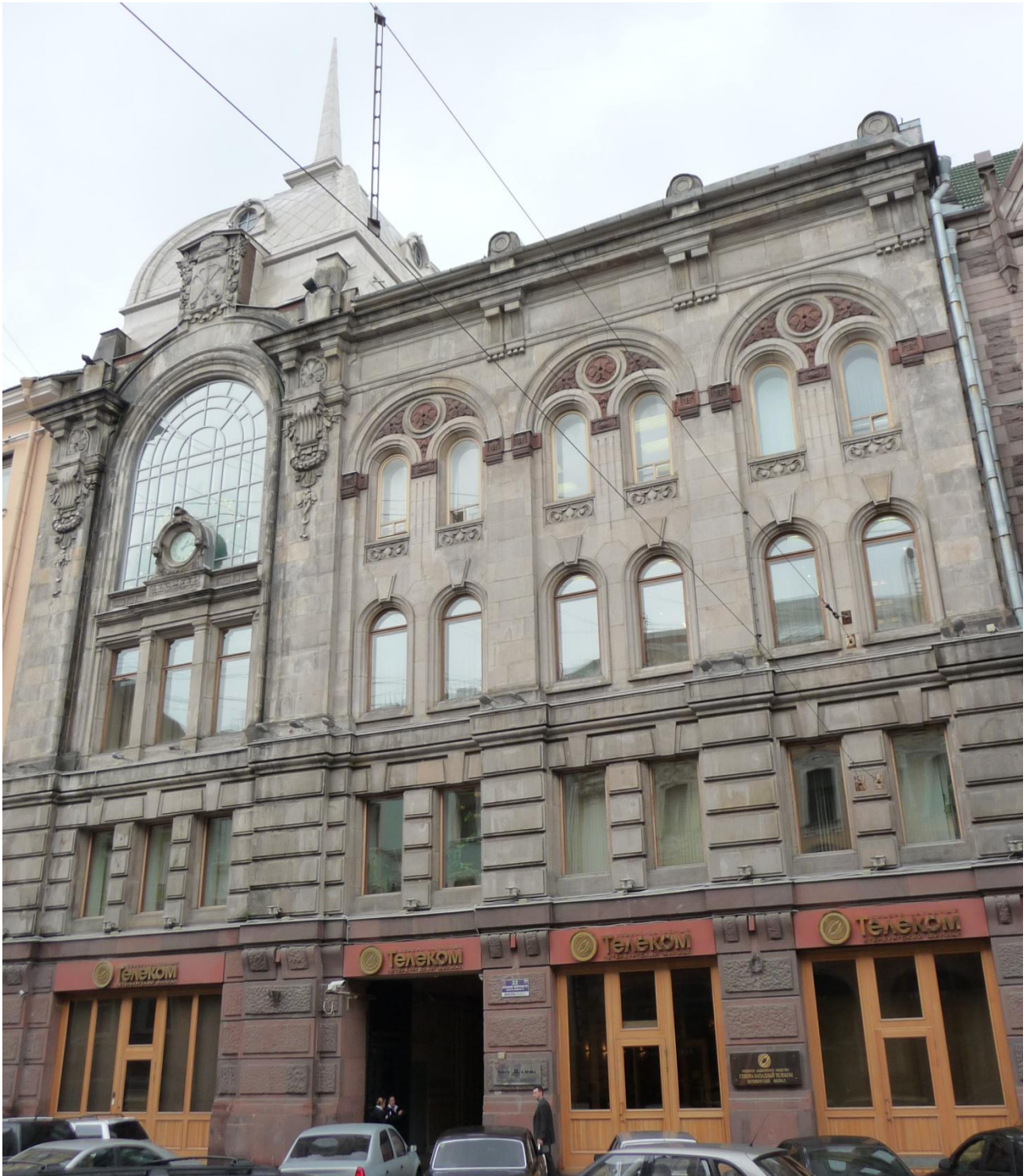
Figure 33. Central Telephone station.
