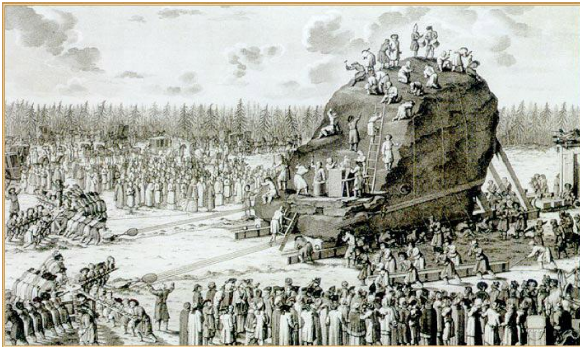
Figure 77 Drawing of the carving of a huge boulder that formed the basement of the statue
