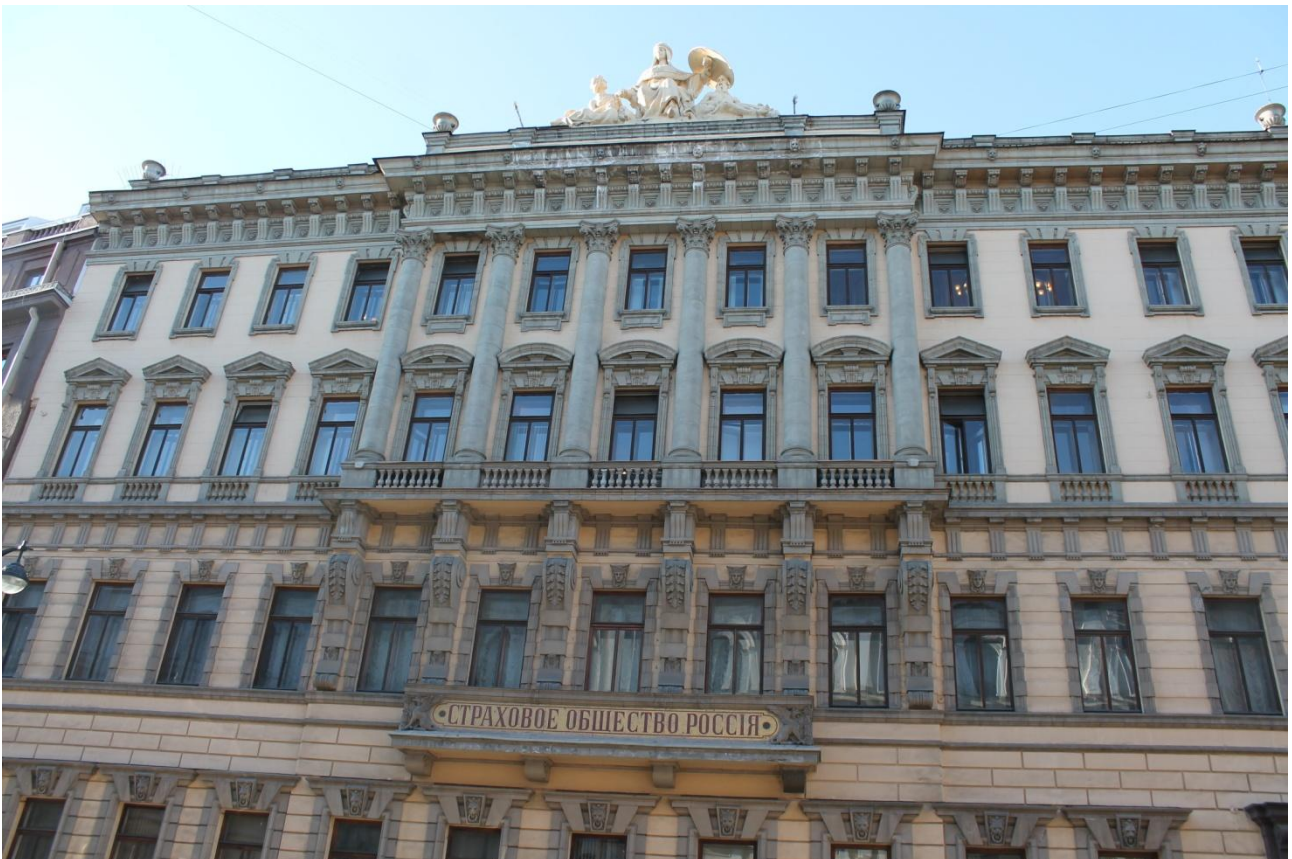
Figure 43 House built for Insurance company “Russia” with red Gangut granite and yellow Württemberg sandstone
