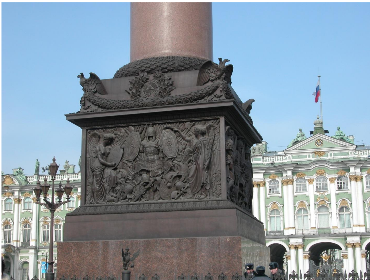
Figure 96 Particular of the basement
