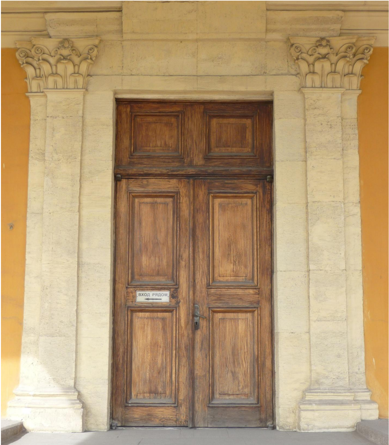
Figure 135 View of the frame of the portal
