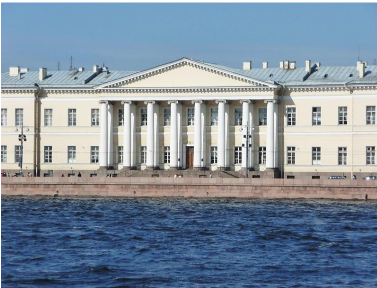
Figure 140 View from the other side of the embankment
