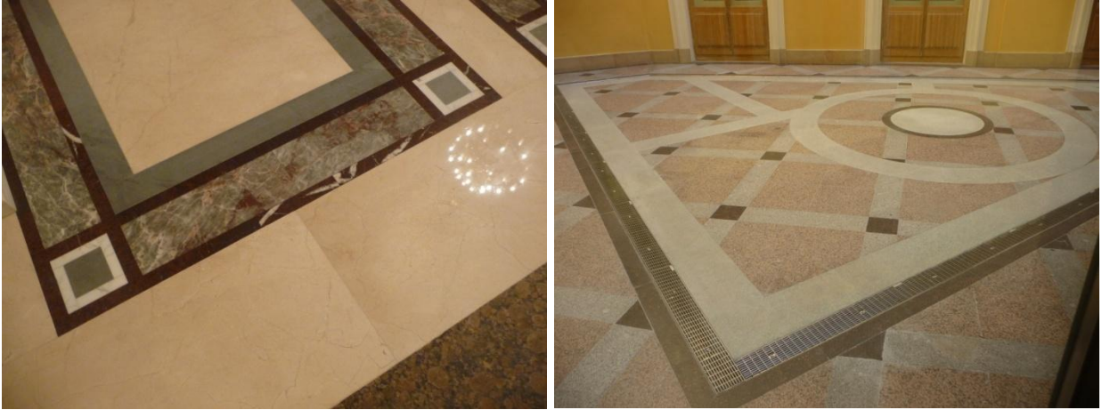
Figure 64 Particulars of the paving
