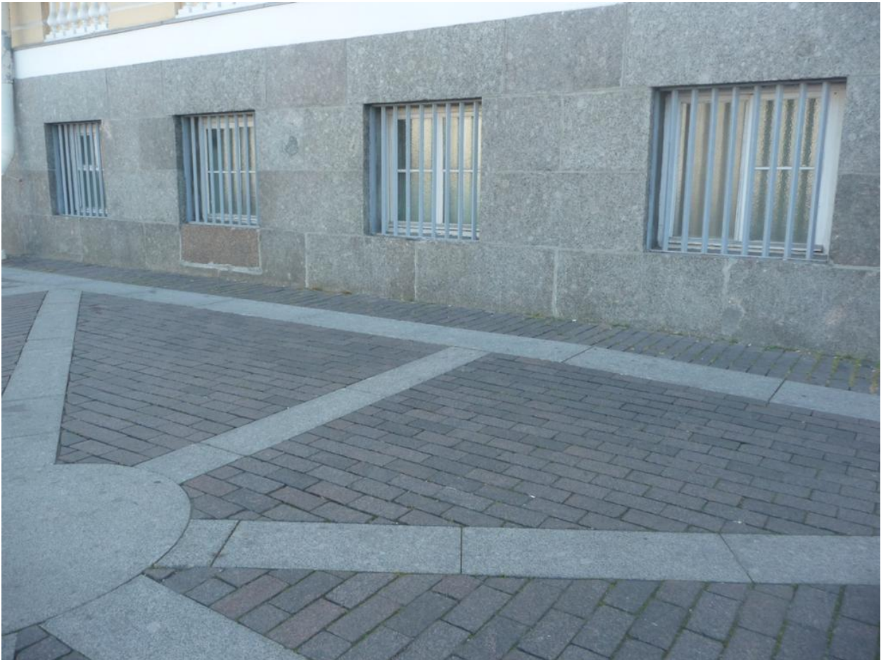
Figure 94 Particular of the basement
