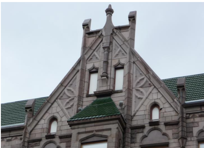
Figure 37. A detail of the front facade in the Faberge's house.
