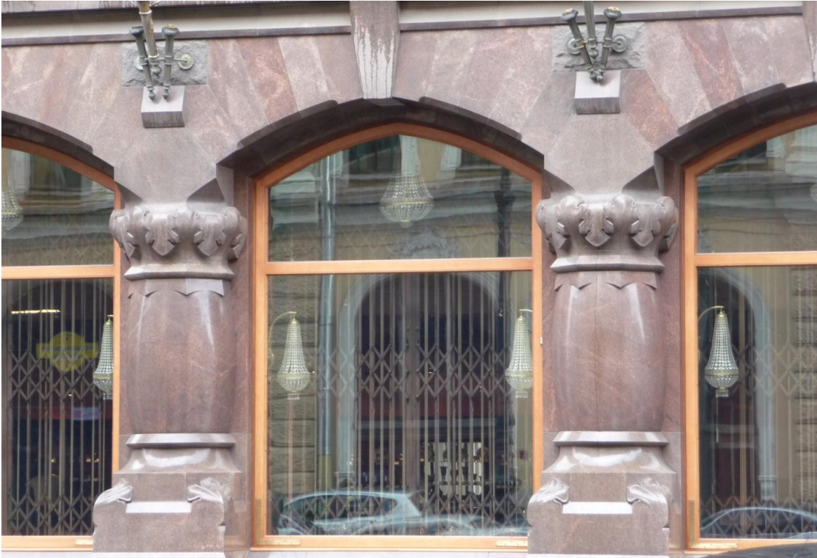
Figure 38. Lower part built from Gangut (Hanko) granite brought from Finland.
