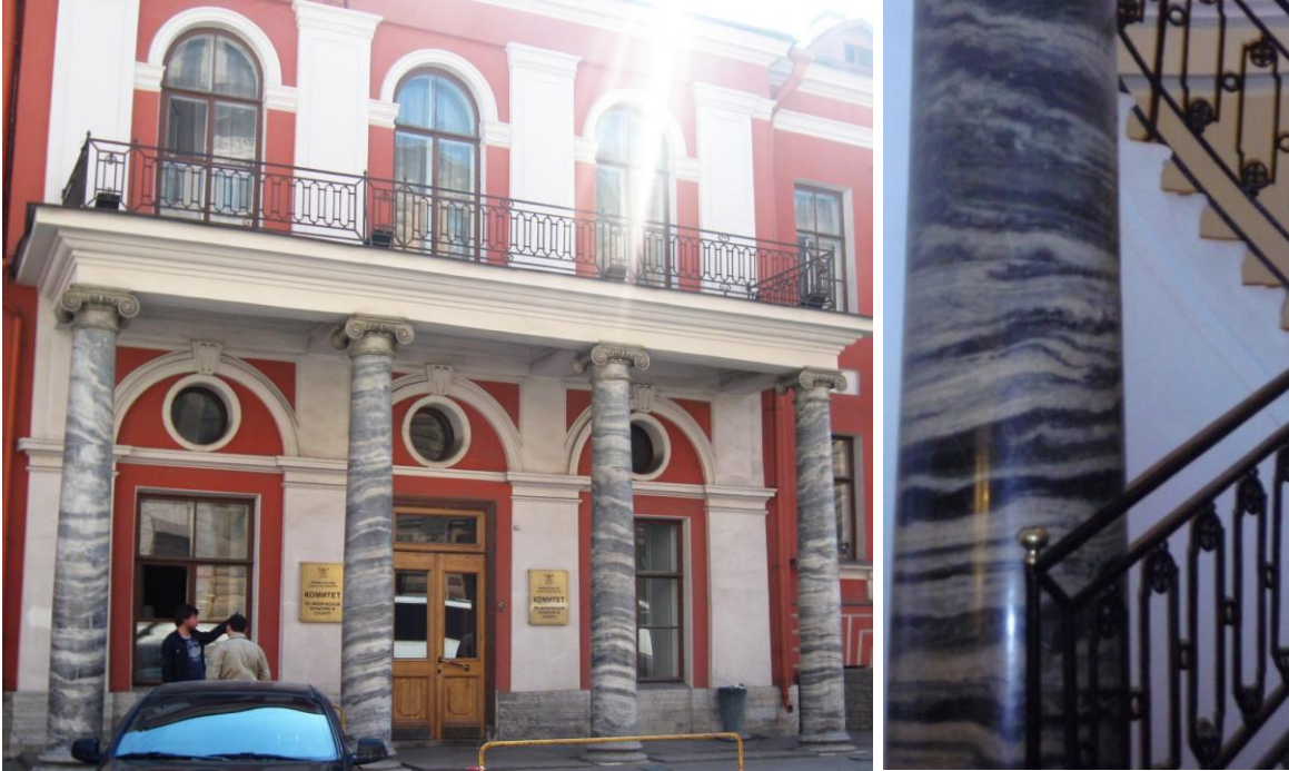
Figure 112 View of the house on the left, and particular of a column on the right- the material used had been Joensuu marble.
