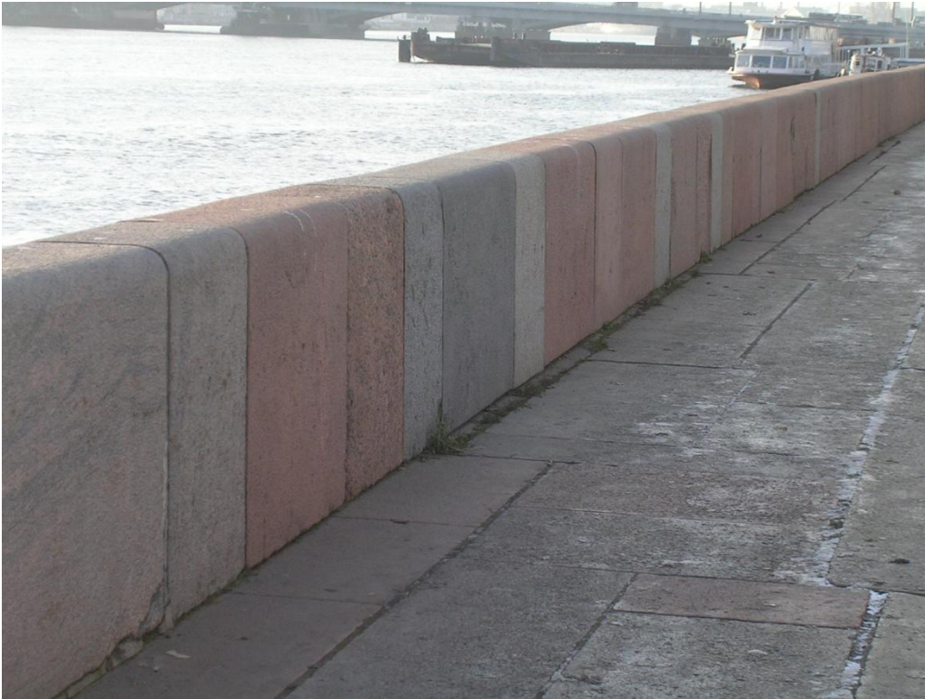
Figure 129 View of the different granites used on the embankment in older times
