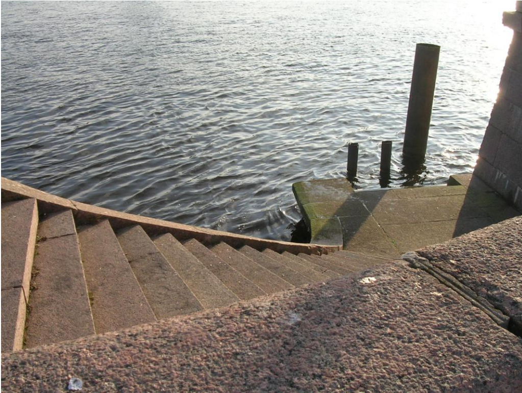
Figure 131 View of the granitic stairs bringing to the pontoon spring-autumn bridge.
