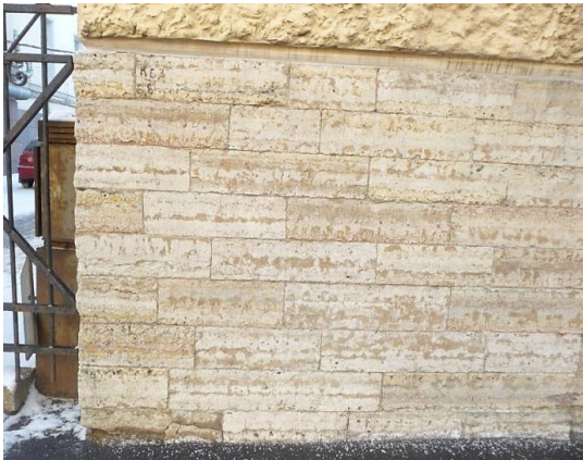
Figure 142 Particular of a base wall in limestone
