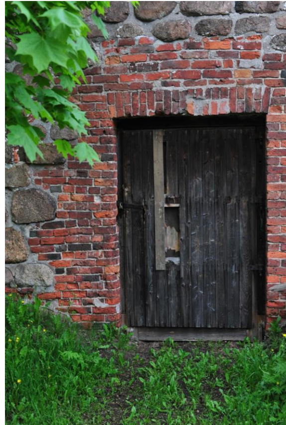
Figure 15. Brick frames on the door opening
