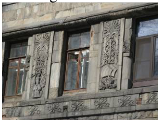
Soapstone (talk-chlorite schist) is used in facing of the first and second floors. The façade of the building is decorated with carved flora and fauna elements. Also, there are carved staffs
