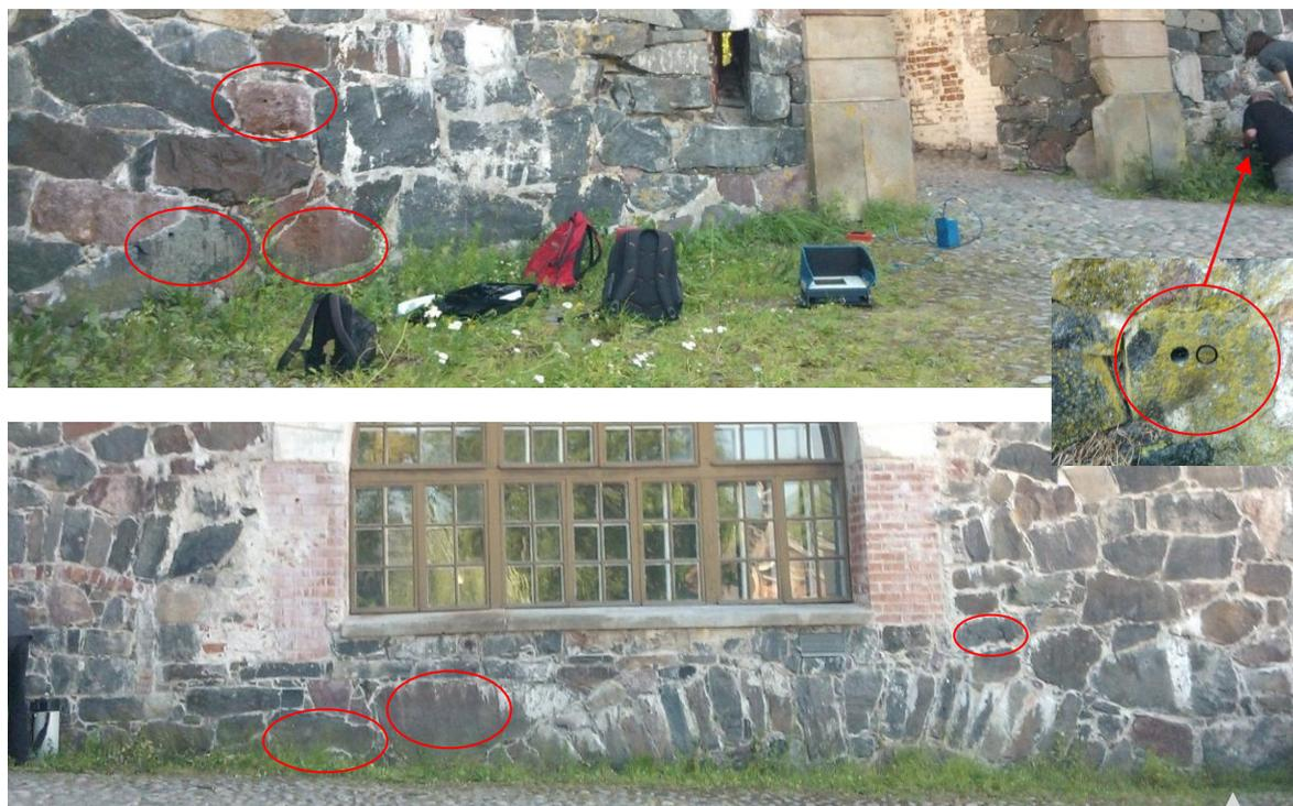
Figure 91. Blocks tested in the upper building of the dry dock
