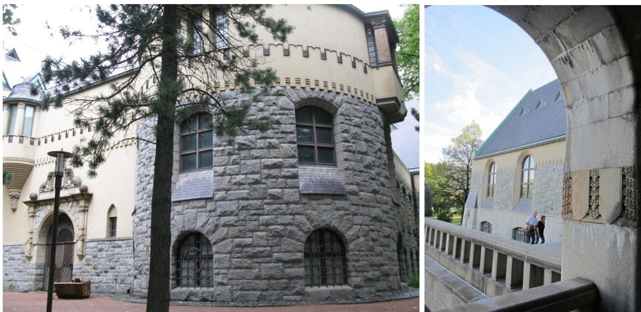
Figure 2. In the figure are shown: the bossy finishing on the main blocks of the façade, the rendered walls and the steatite decorations, and the slate roofs. (Photo: N.Luodes)
