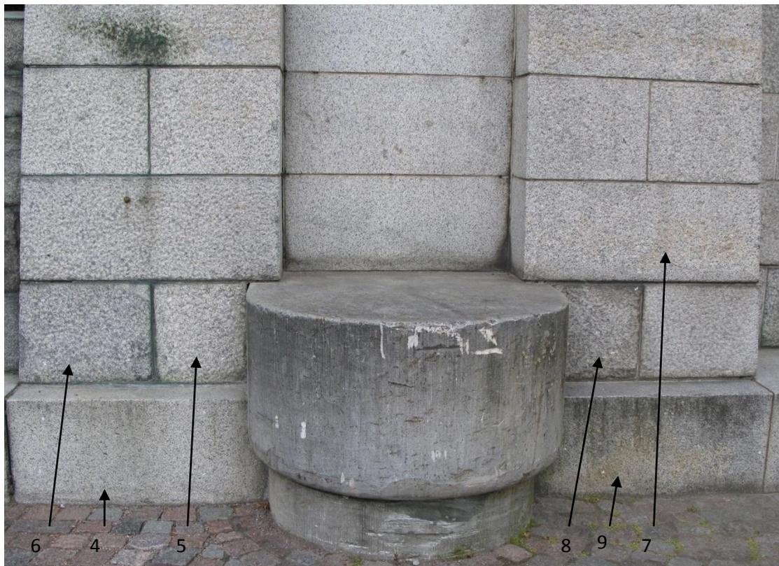
Figure 85 Schmidt hammer on blocks bush hammered facing East
