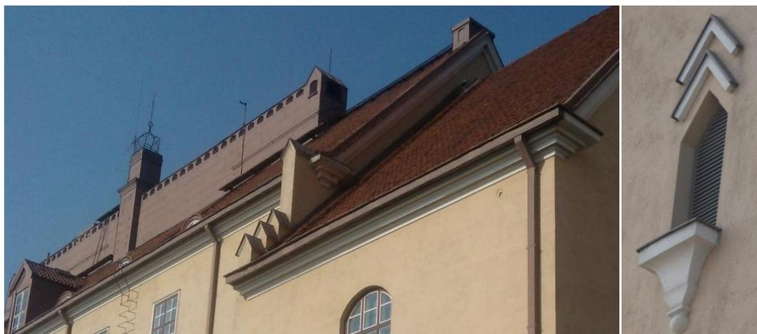
Figure 3. Roof detail from East side. Are visible the dormers, the wall over the ridge of the roof and the architectonic decorative details (on the right). (Photo N. Luodes, GTK)
