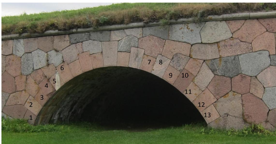
Figure 80 Position of the blocks tested over the left arc of the Tenaille. (Photo: H.Pirinen)
