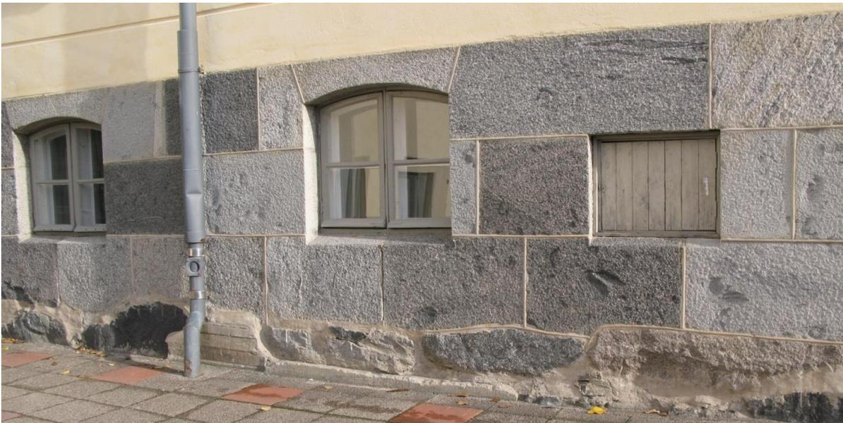
Figure 6. Inner yard enlargement dated 1940, showing heterogeneous material.
