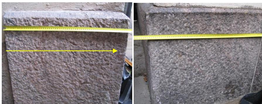
Figure 56. Corner block measures and line of measurements. (photo: N.Luodes)
