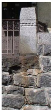
Changes of colour determined by leaching of material in contact with the stone could be noticed in the stair parapet as visible from Figure 12.
