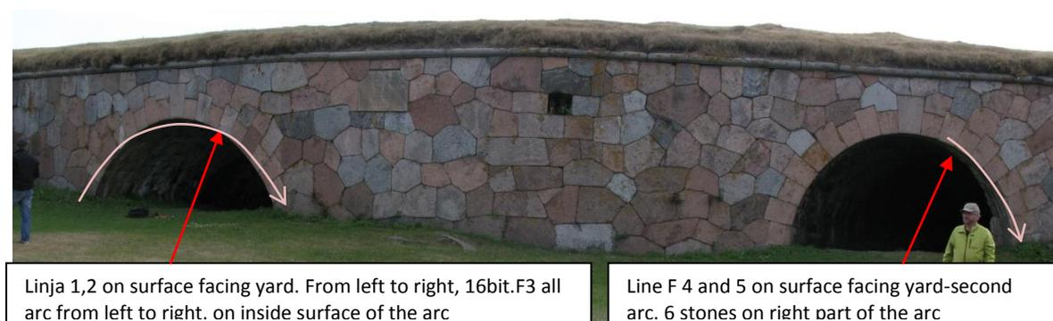
Figure 69 Position of the GPR measurement lines over the Tenaille in Kustaanmiekkä.
