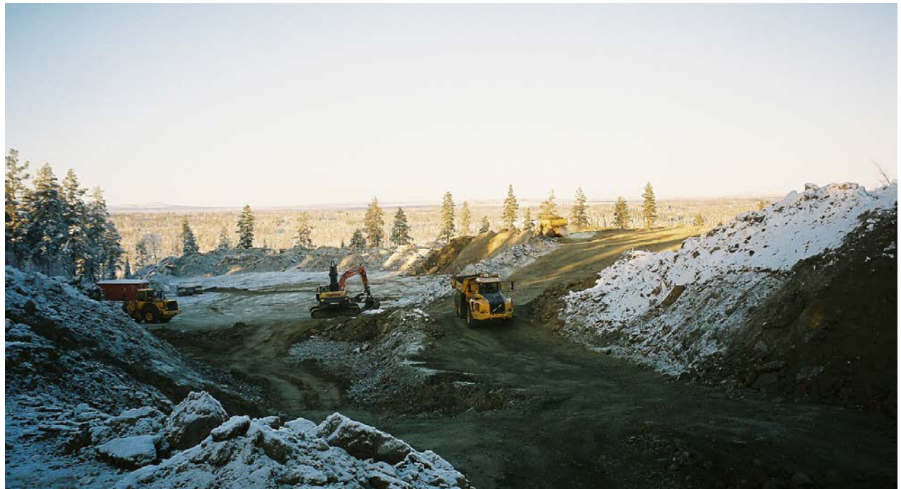
Figure 11. Working the ground to prepare for mining in Kaunisvaara, Pajala. Foto: Niclas Dahlström.
