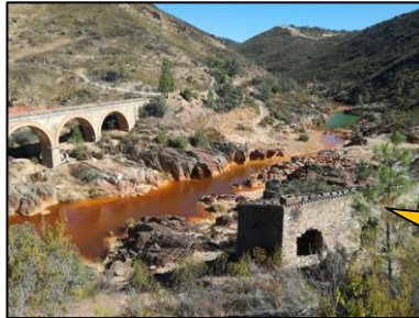
Absence of control measures
